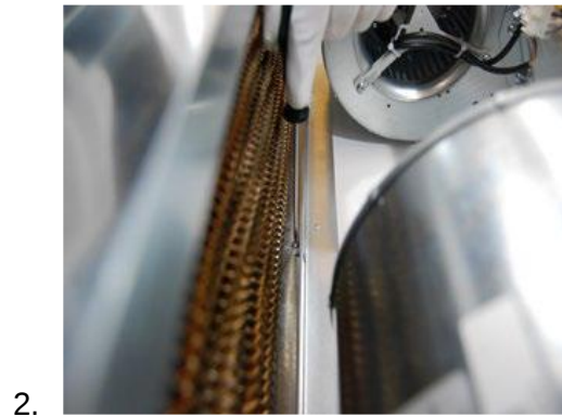
Drain Plug at the Main Collector
